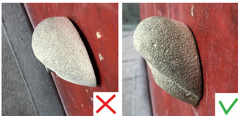
Picture 9. All the edges need to be well attached to the wall
