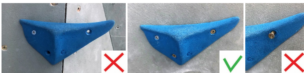
Picture 10. All the edges need to be well attached to the wall, assembling screws have to be screwed to the stop
